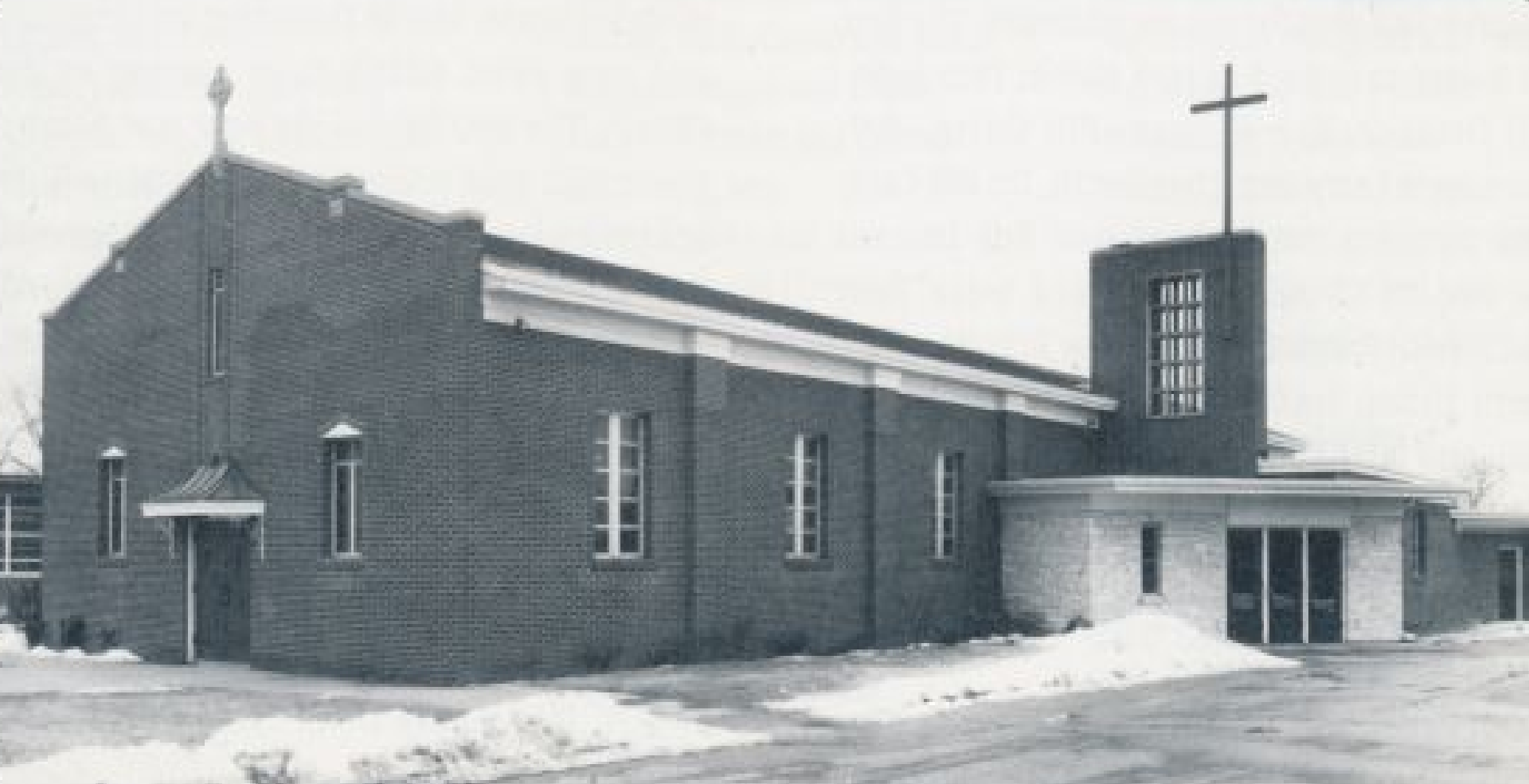
The original church after a remodeling, renovation and an extension.
