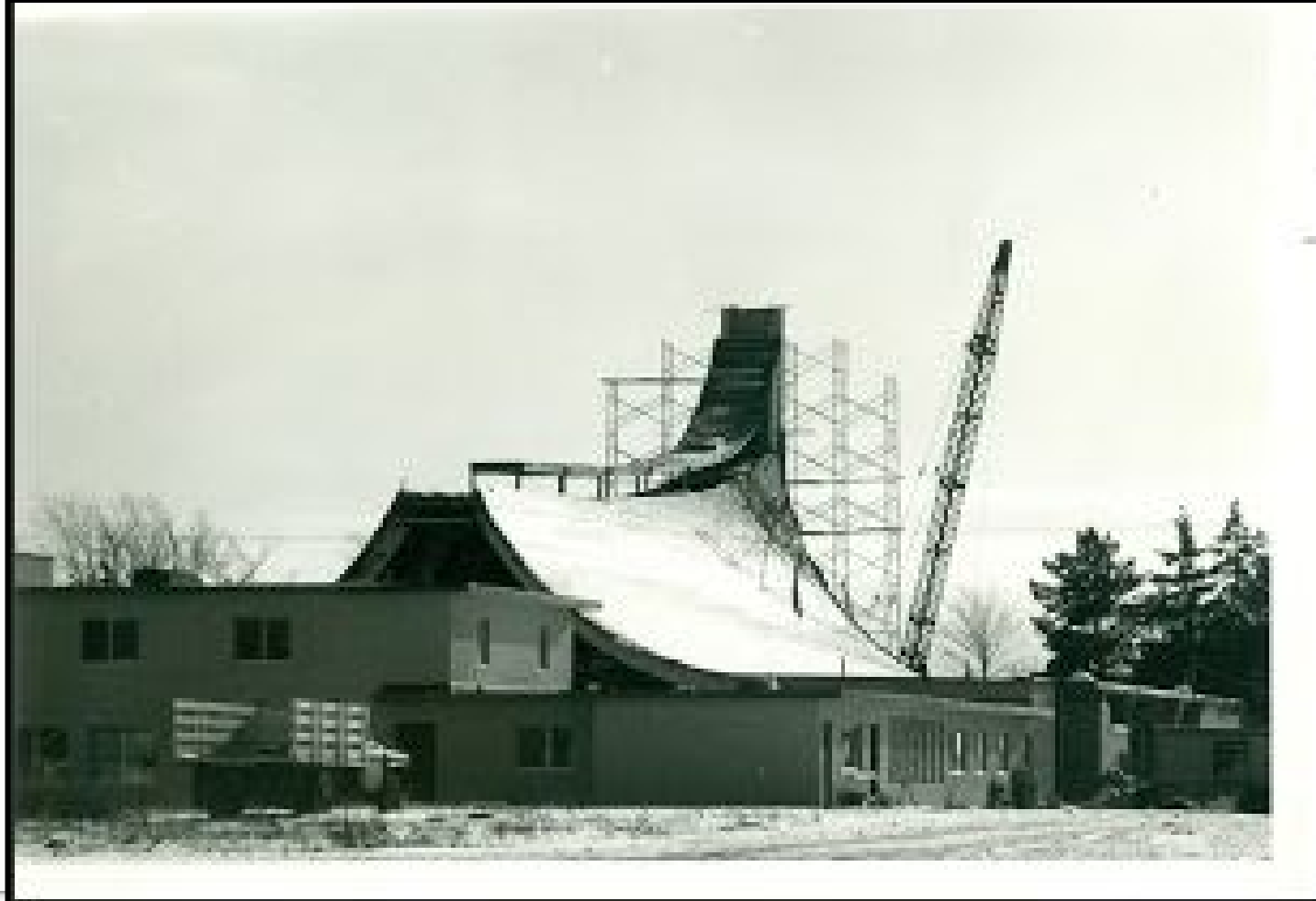
The church, rectory and parish office after roofing was installed in 1966.
