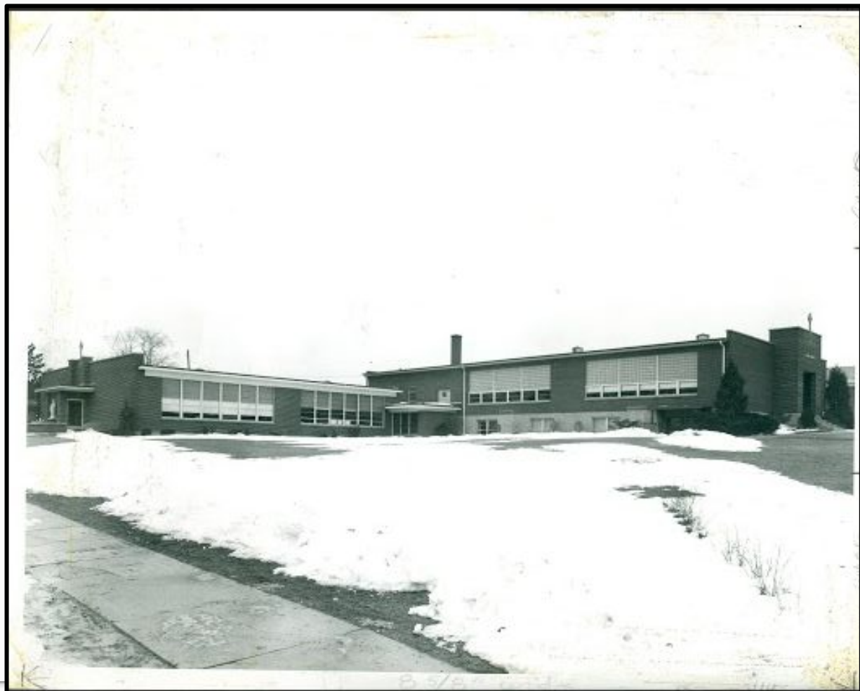
IHM School after the original four-classroom section and two additions.
